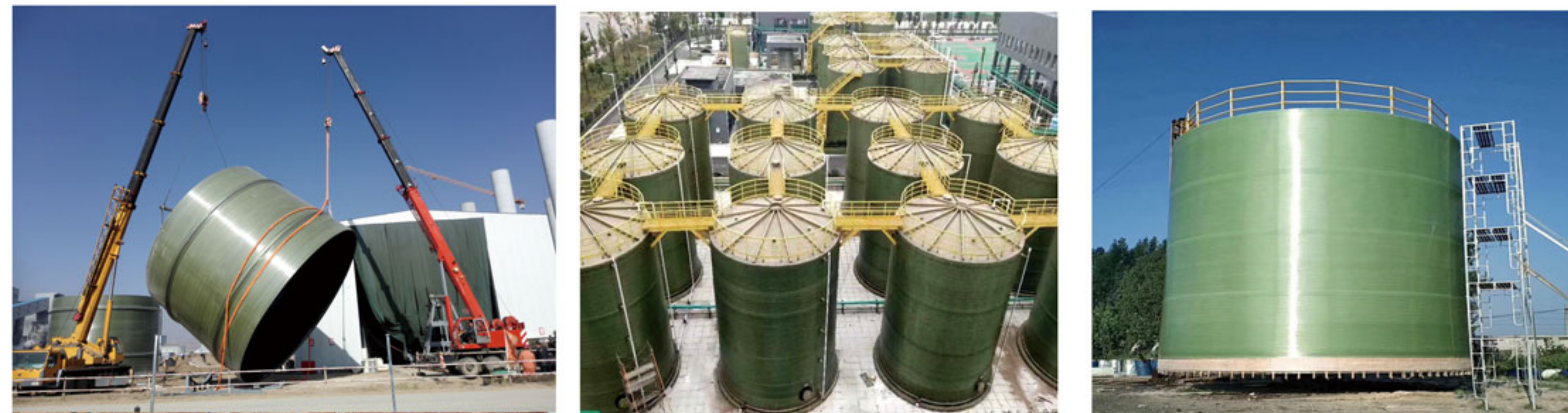
现场缠绕大型罐 SITE WINDING MAX TANK
